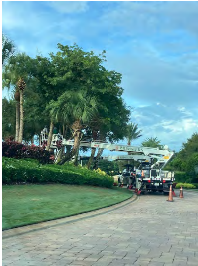
(7) Holiday Lighting Installation
