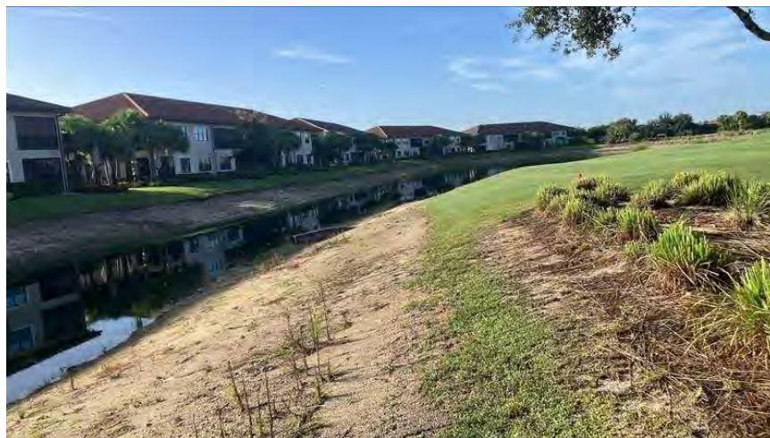
Figure 7-20/21b. Existing shoreline condition at Lake 20/21, opposite view.
