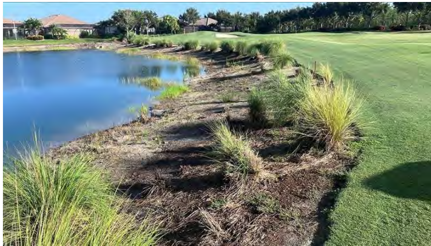
Figure 7-8a. Existing shoreline condition at Lake 8.
