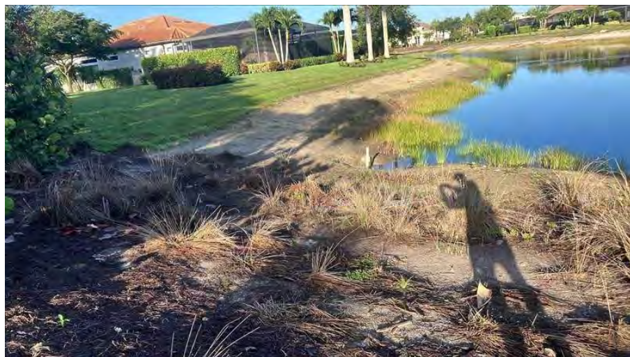
Figure 7-14b. Existing shoreline condition at Lake 14, opposite view.
