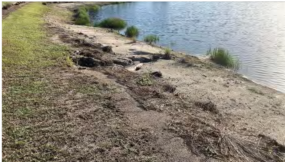
Figure 7-24b. Existing shoreline condition at Lake 24, opposite view.
