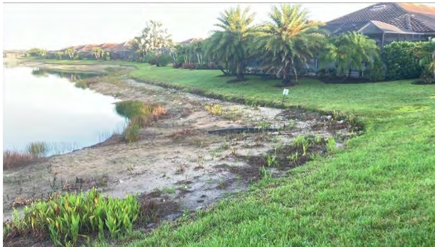
Figure 7-17a. Existing shoreline condition at Lake 17.
