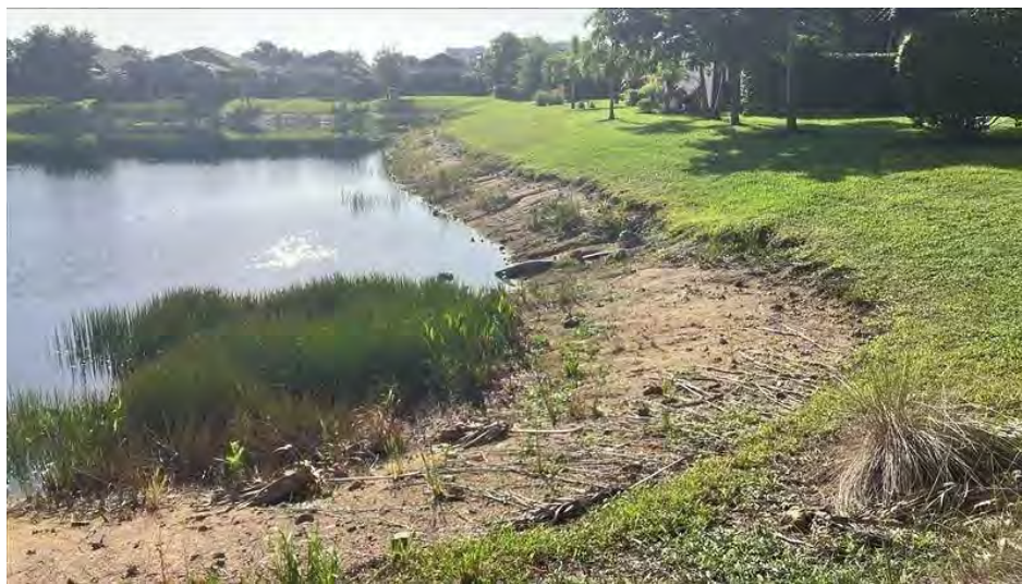
Figure 7-26a. Existing shoreline condition at Lake 26.
