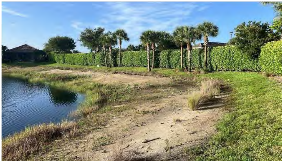
Figure 7-18/19a. Existing shoreline condition at Lake 18/19.
