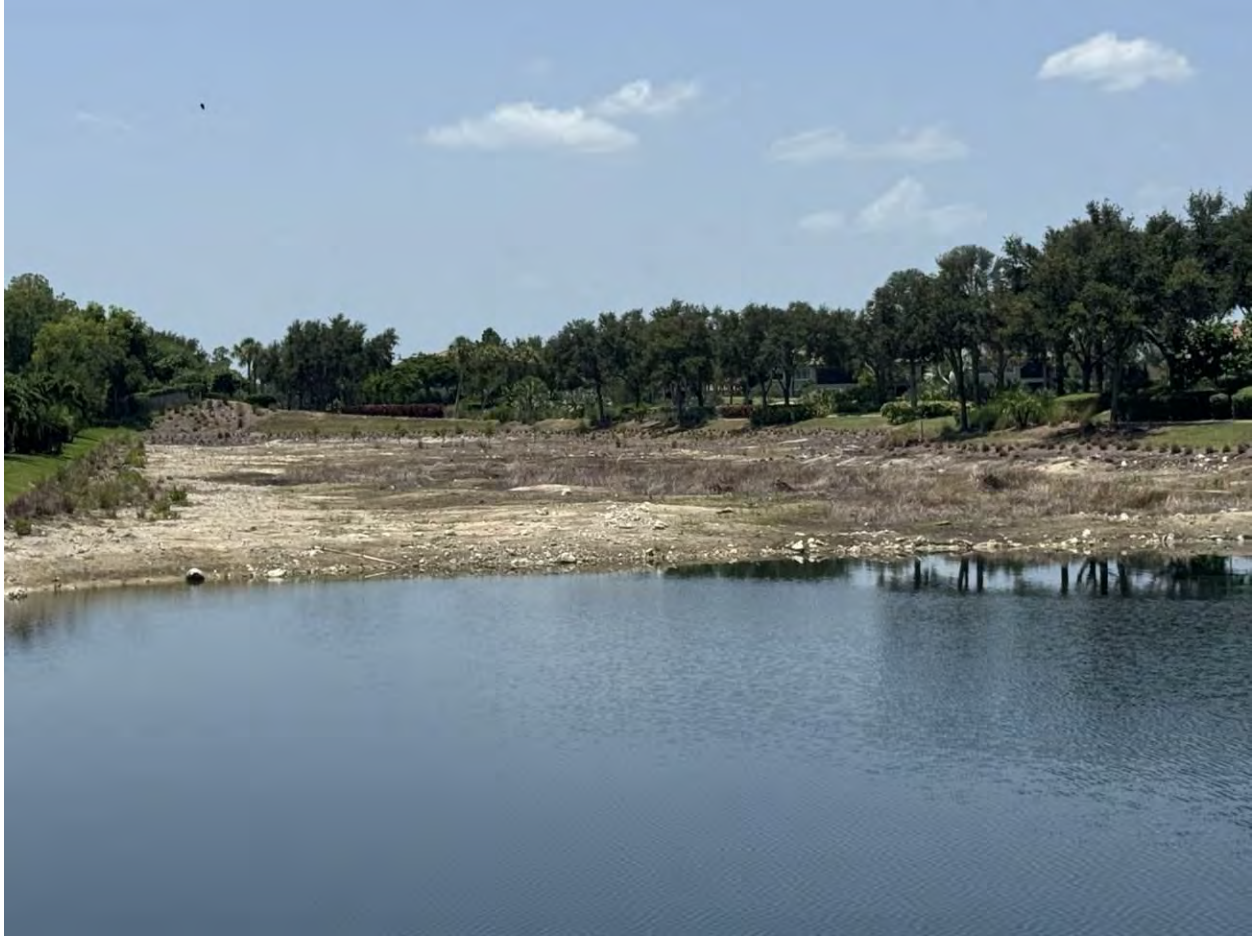
Figure 7-11b. Existing shoreline condition at Lake 11, opposite view, showing the exposed lake bottom and remnant stumps during low water, with newly installed littoral plantings along the upper bank.
