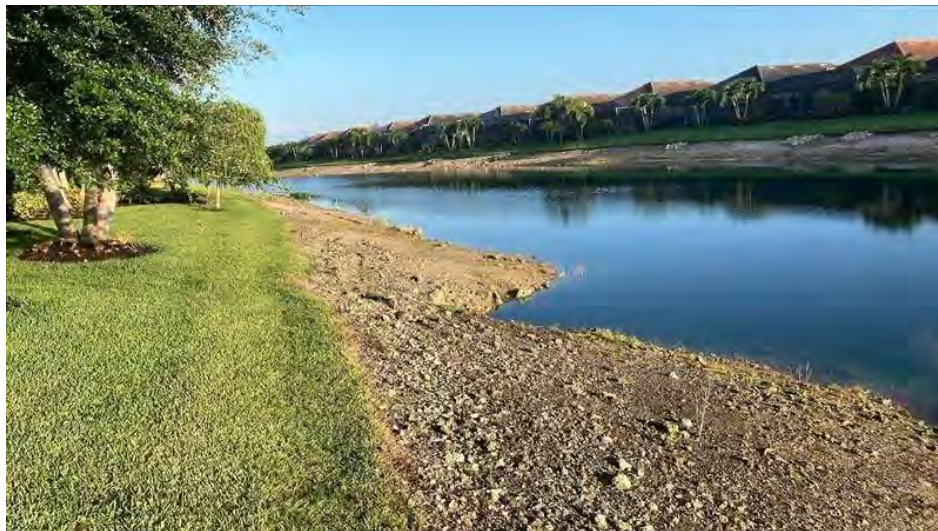
Figure 7-22b. Existing shoreline condition at Lake 22, opposite view.
