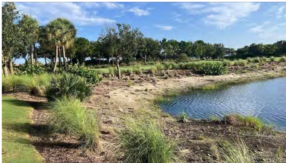
Figure 7-23b. Existing shoreline condition at Lake 23, opposite view.
