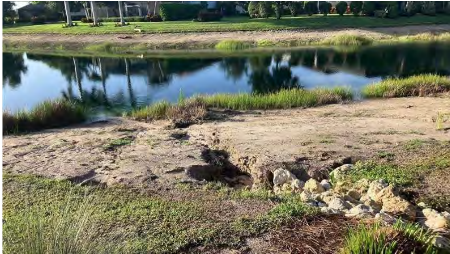
Figure 7-14a. Existing shoreline condition at Lake 14.
