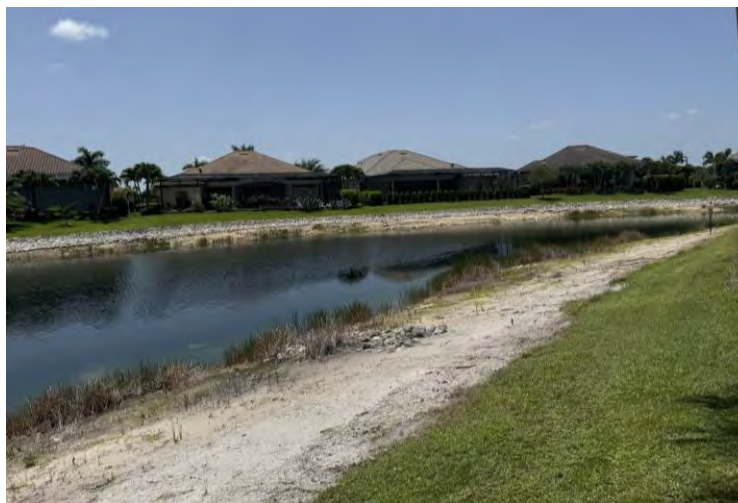
Figure 7-12b. Existing shoreline condition at Lake 12, opposite view, showing the riprap-armored shoreline and sandy bank near the designated littoral shelf planting area.
