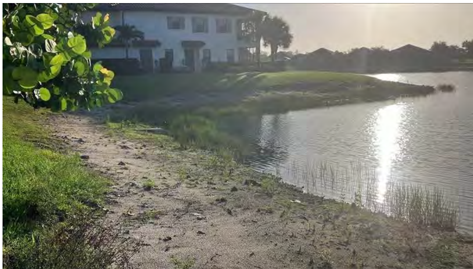
Figure 7-18/19b. Existing shoreline condition at Lake 18/19, opposite view.
