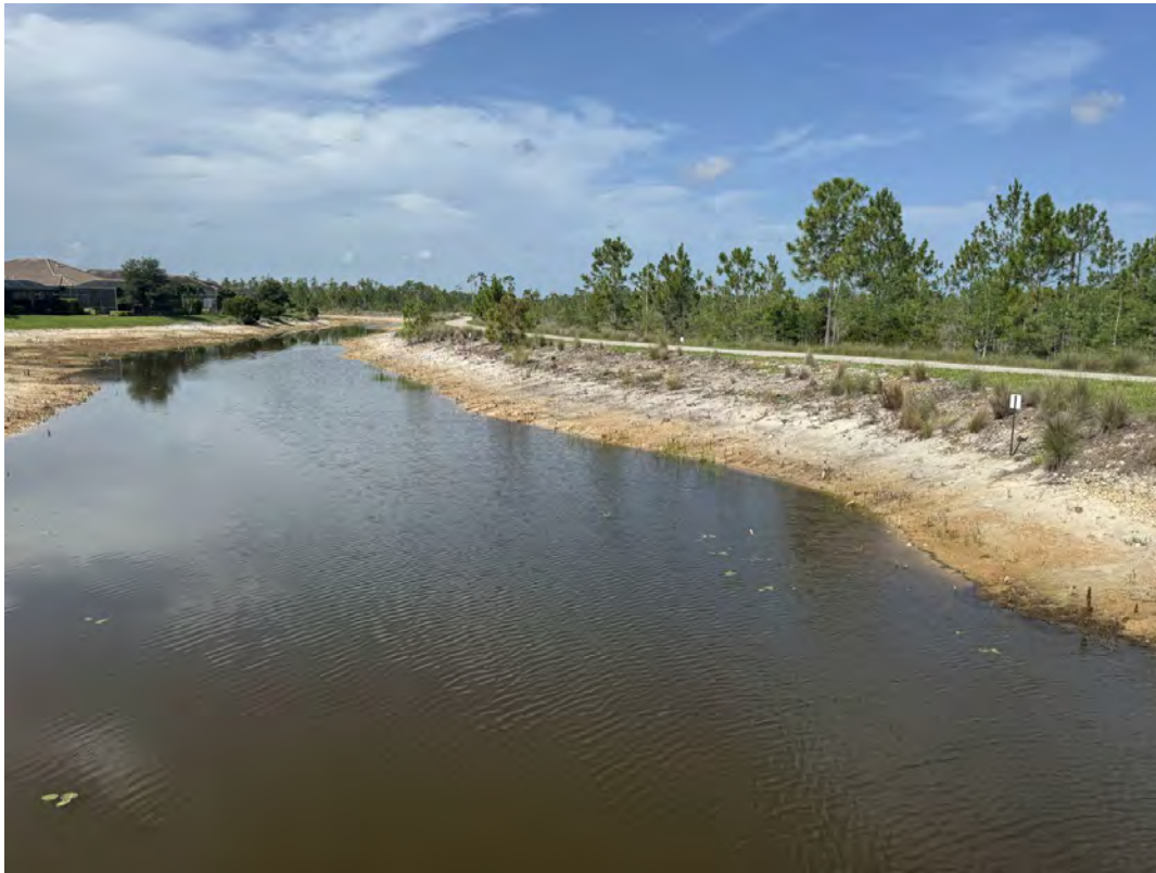
Figure 7-28a. Existing shoreline condition along the Flow Way Channel, showing the sandy bank and open water fronting the adjacent walking path.
