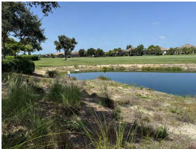
Figure 7-4a. Existing shoreline condition at Lake 4, showing the sandy bank and fairway edge with scattered cordgrass clumps along the water's edge.
