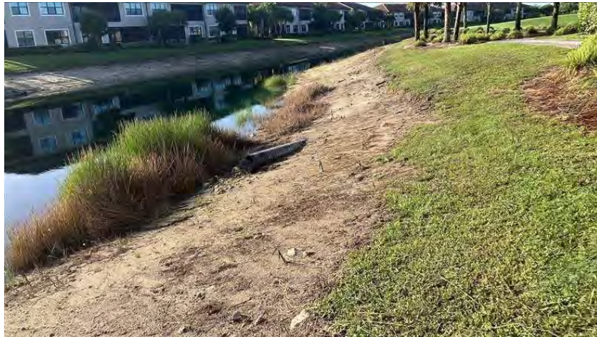
Figure 7-20/21a. Existing shoreline condition at Lake 20/21.
