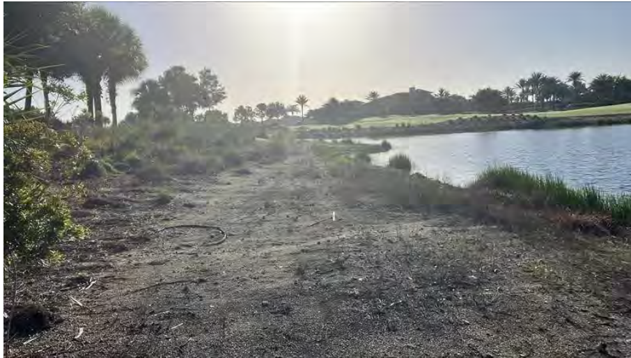
Figure 7-24a. Existing shoreline condition at Lake 24.
