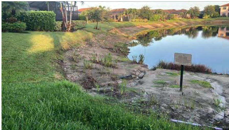
Figure 7-16a. Existing shoreline condition at Lake 16.
