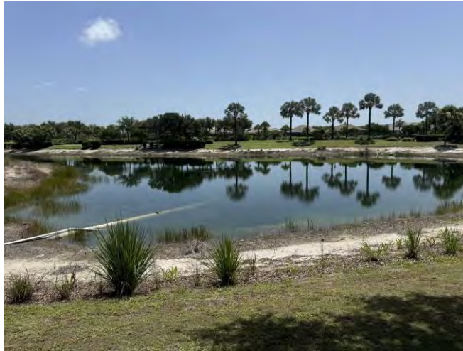
Figure 7-10a. Existing shoreline condition at Lake 10, showing exposed sandy bank fronting residential lots with an isolated drainage pipe partially submerged at the shoreline.
