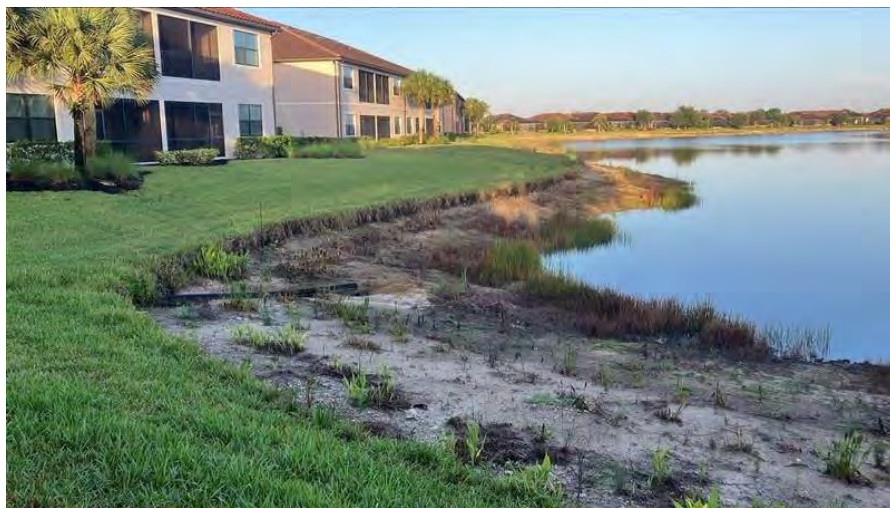
Figure 7-17b. Existing shoreline condition at Lake 17, opposite view.
