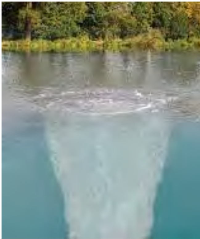
Figure 6-3c. Reference photo (not Flow Way) of a subsurface aeration system in operation, showing the circulation pattern created at the water surface.
