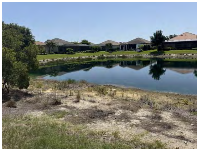
Figure 7-3b. Existing shoreline condition at Lake 3, opposite view, showing the exposed sandy shelf transitioning to maintained turf.
