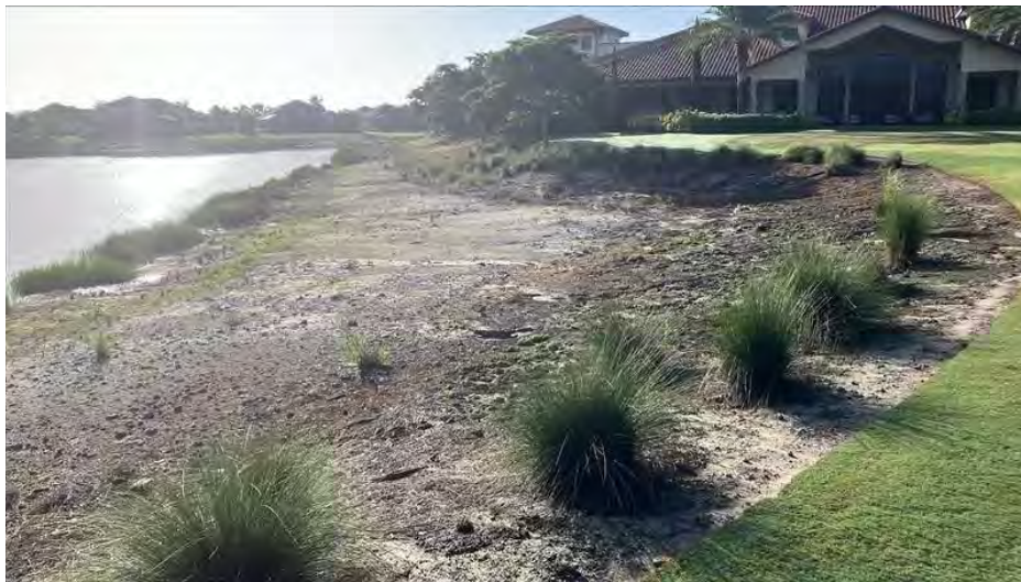
Figure 7-23a. Existing shoreline condition at Lake 23.
