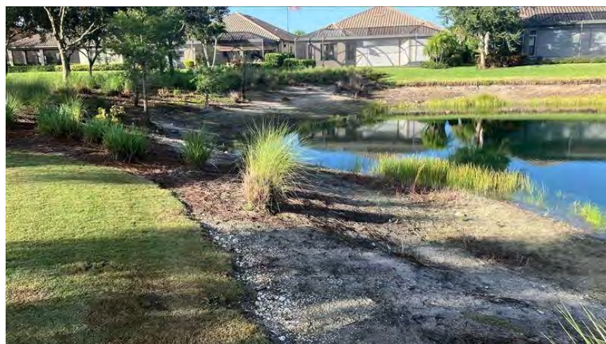
Figure 7-8b. Existing shoreline condition at Lake 8, opposite view.
