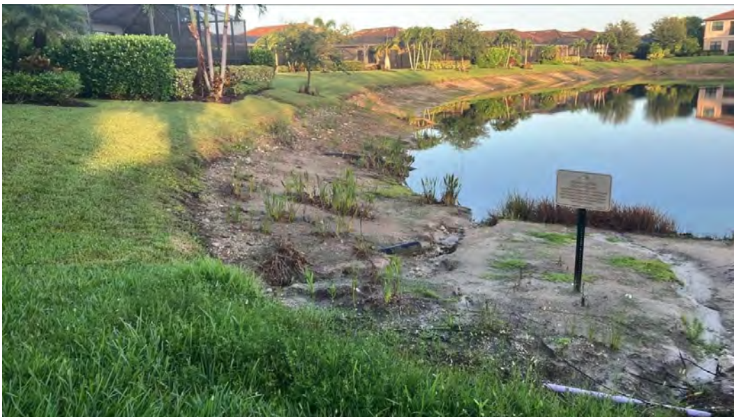
Figure 4-2. Exposed pipe within a designated littoral shelf planting area, immediately adjacent to District signage. Littoral plantings in this reach are sparse and struggling on a disturbed, unstabilized bank.
