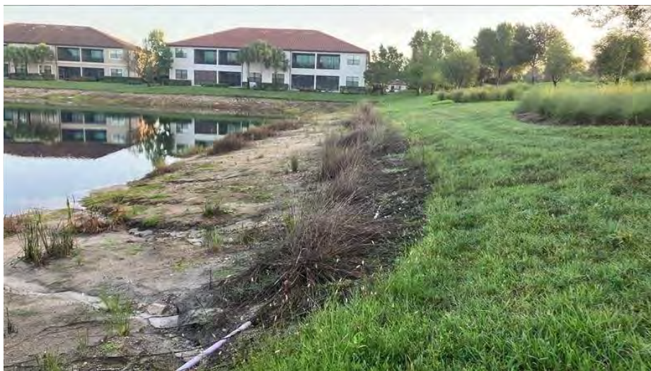
Figure 7-16b. Existing shoreline condition at Lake 16, opposite view.
