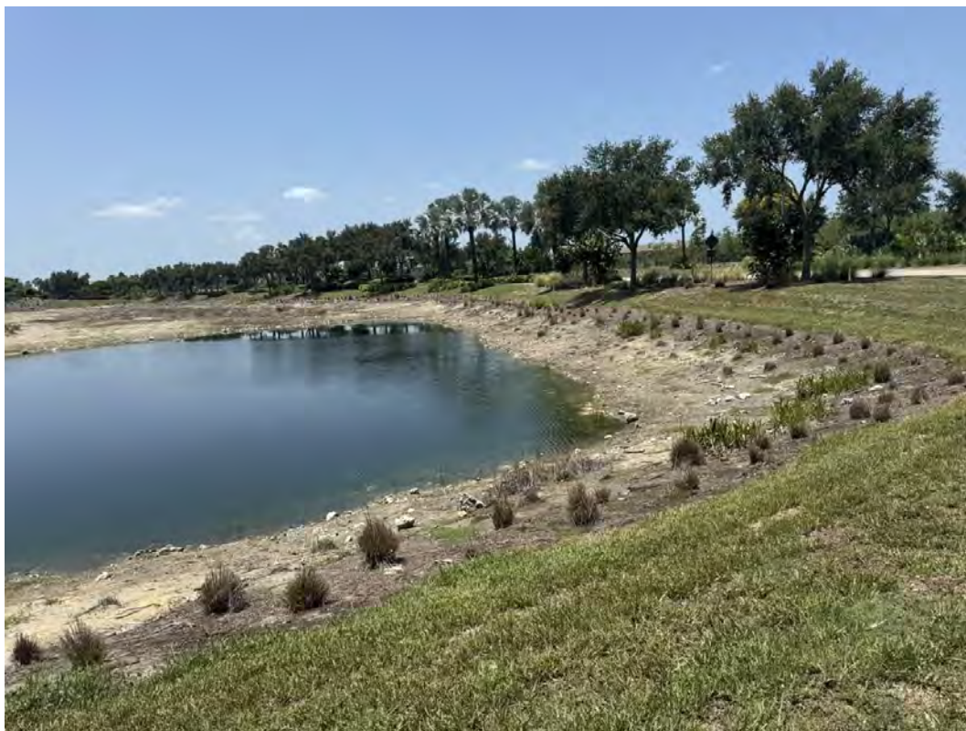
Figure 7-11a. Existing shoreline condition at Lake 11, showing low water levels exposing a wide bare bank with scattered cordgrass clumps along the perimeter.
