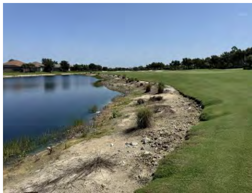
Figure 7-2b. Existing shoreline condition at Lake 2, showing sparse, isolated grass clumps on an eroded, rocky shoreline with limited continuous littoral coverage.
