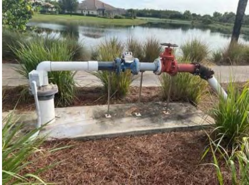
(8) Irrigation System Repair
