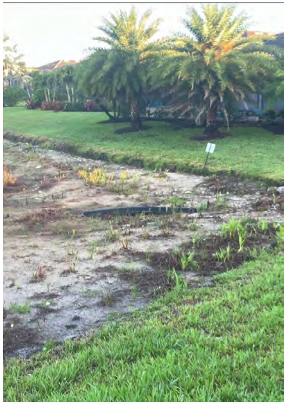
Figure 4-6. Exposed pipe run through an area of sparse, patchy littoral establishment — illustrating the link between disturbed piping and failed plantings.
