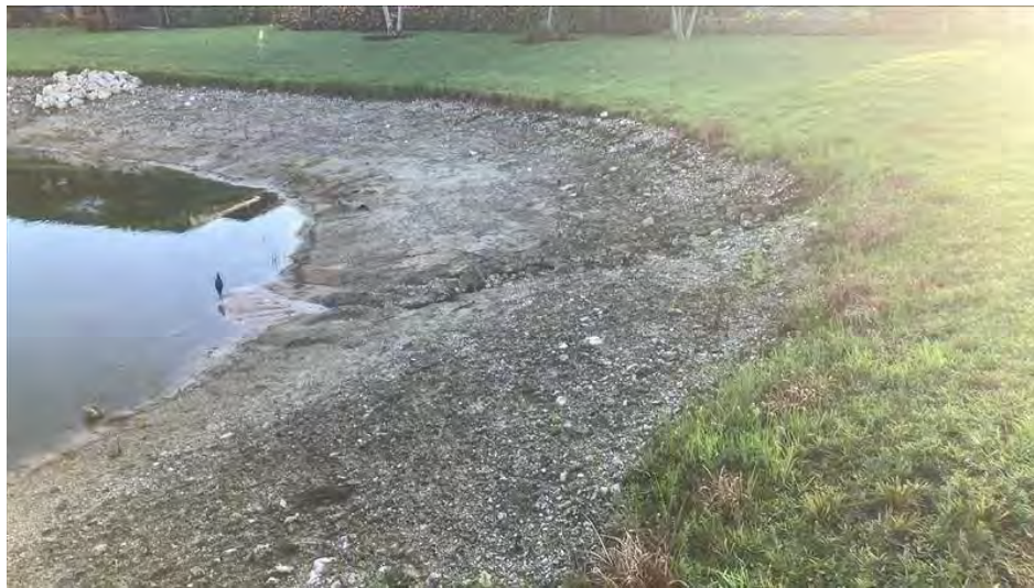
Figure 7-22a. Existing shoreline condition at Lake 22.
