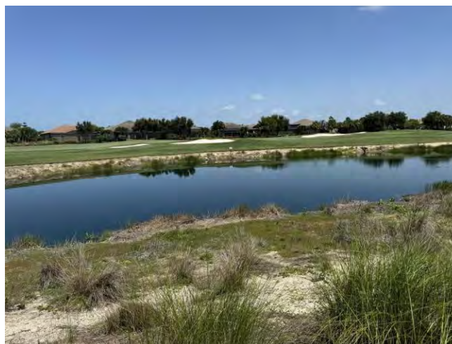
Figure 7-4b. Existing shoreline condition at Lake 4, opposite view, showing the exposed sandy littoral shelf fronting the green and bunker complex.
