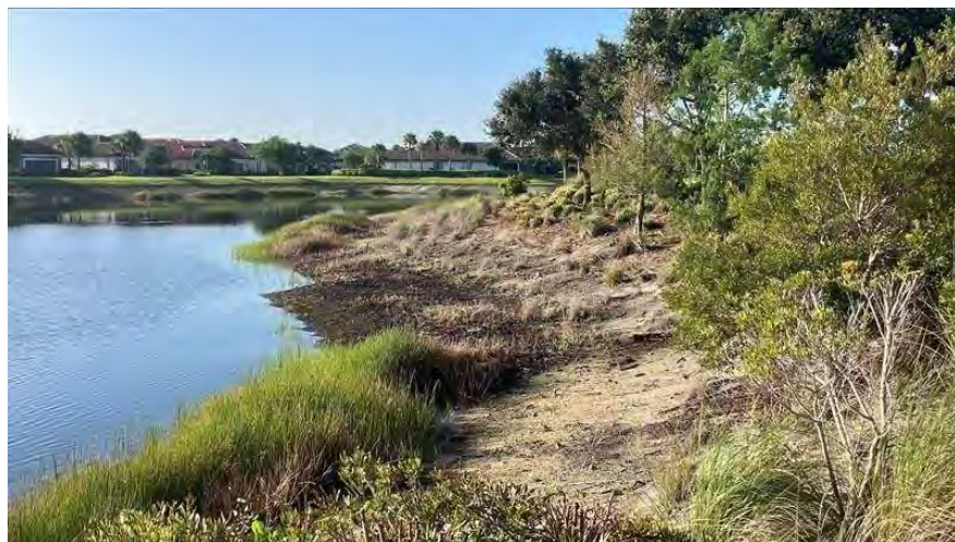
Figure 7-25b. Existing shoreline condition at Lake 25, opposite view.
