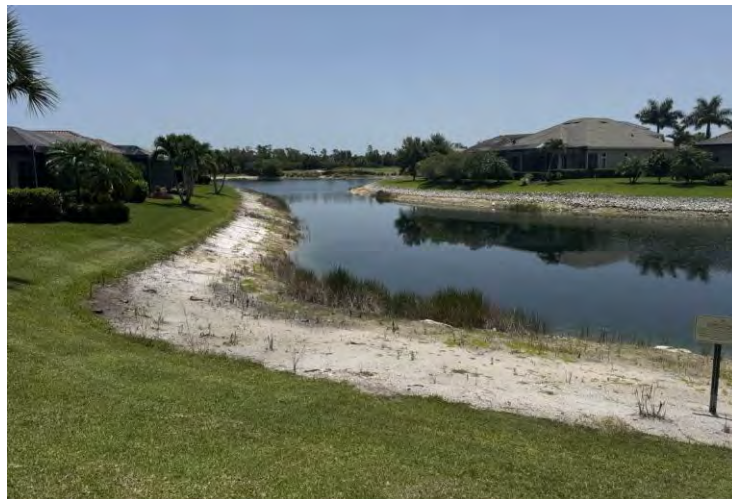
Figure 7-12a. Existing shoreline condition at Lake 12, showing a riprap-stabilized bank fronting residential lots with sparse littoral vegetation at the shoreline.
