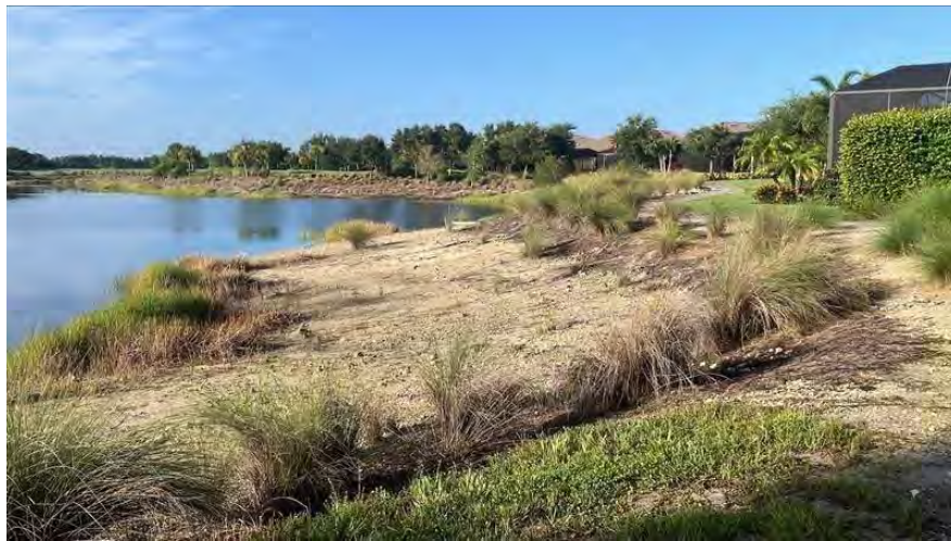
Figure 7-25a. Existing shoreline condition at Lake 25.
