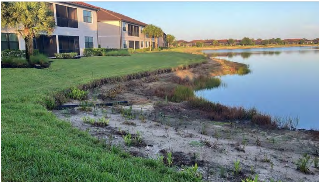
Figure 4-3. Separated pipe run lying loose on the shelf. Sections have pulled apart at the joints and shifted out of alignment — the characteristic signature of repeated flotation under high-water conditions.
