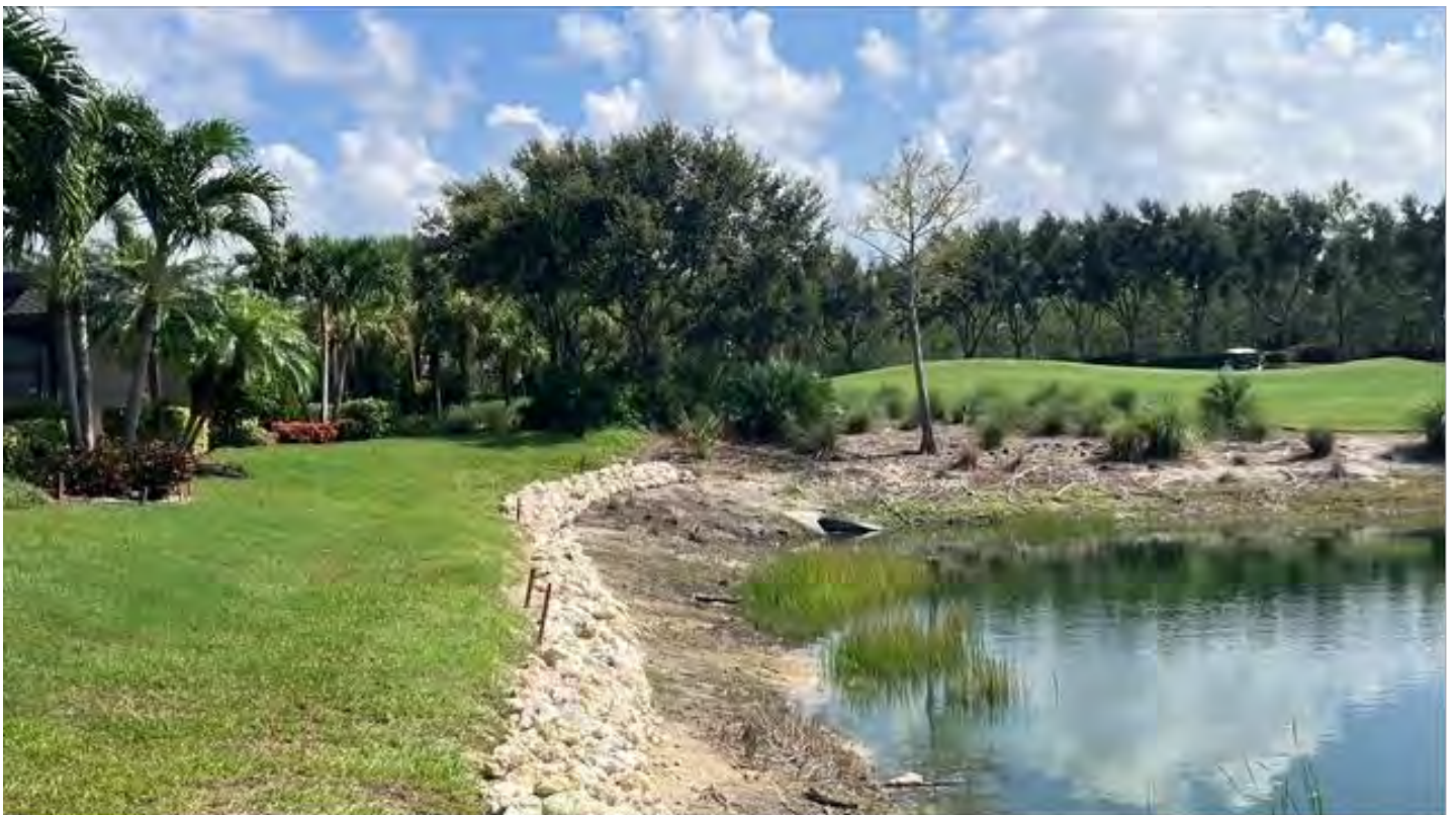
(5) RipRap Repair on Lake 8
