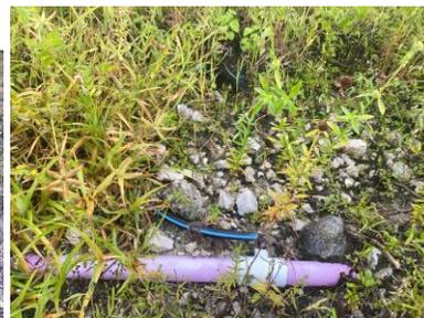
**Sprinkler laying down causing washout**
