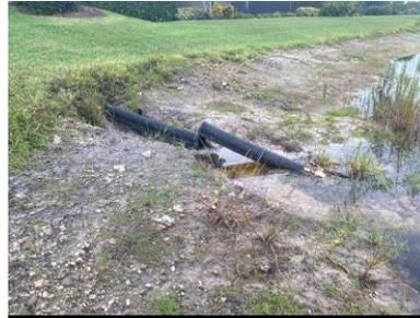
**Drainage pipe broke causing washout**
