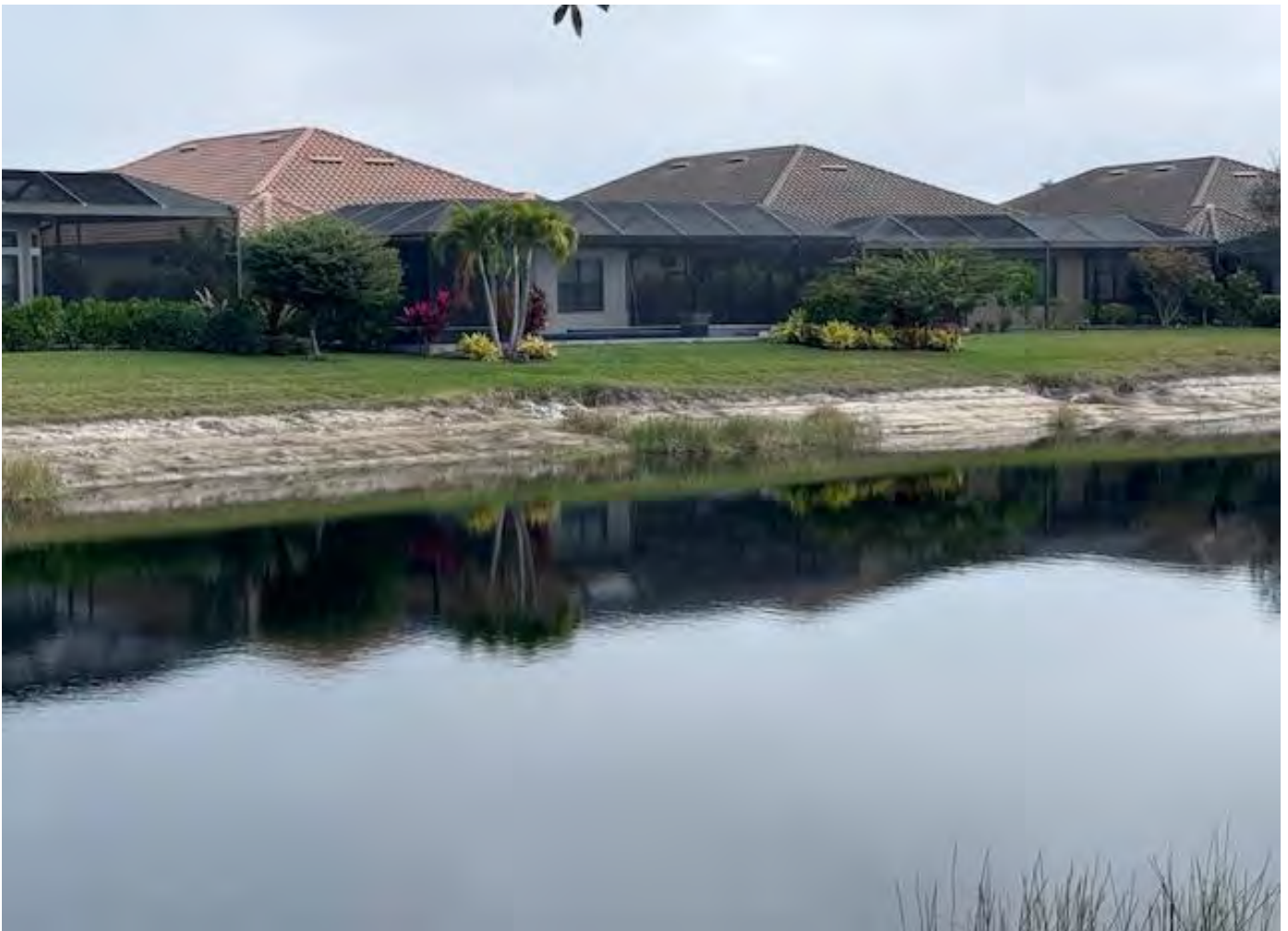
(4) Erosion repairs Lake 14 FY 26 CIP
