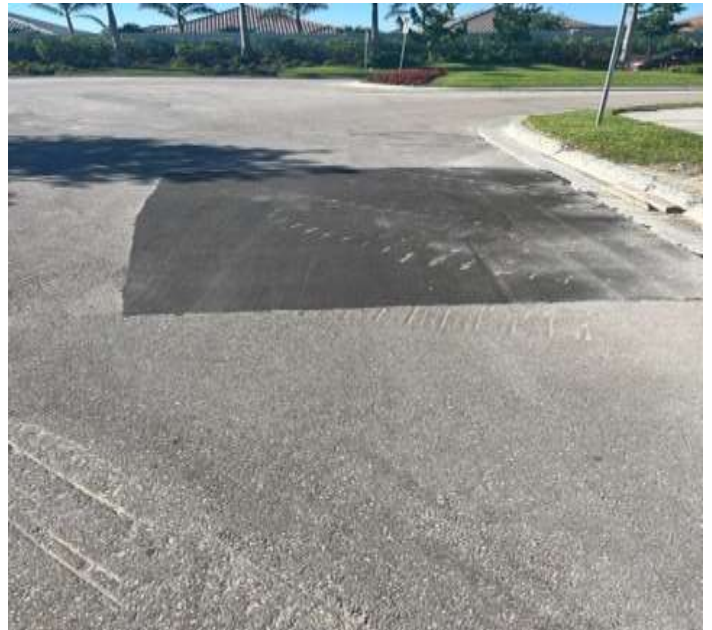
Pothole replaced on Center Place Blvd.
