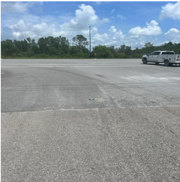
After sand was cleaned up on Center Place Boulevard.
