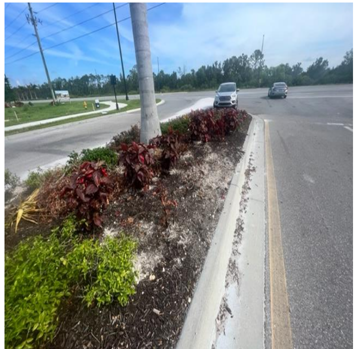
Median in Center Place Boulevard before it was restored.
