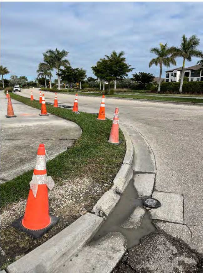
Before replacing curb and gutter on Center Place Blvd.
