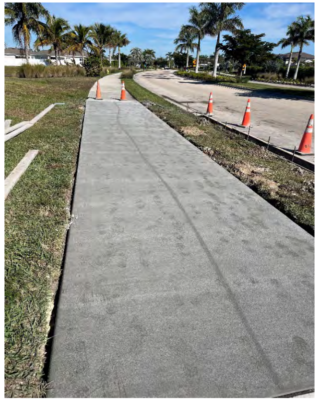
Completion of sidewalk on Center Place Blvd.
