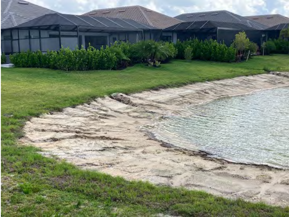
Erosion issues; scheduled installation of littoral plantings
