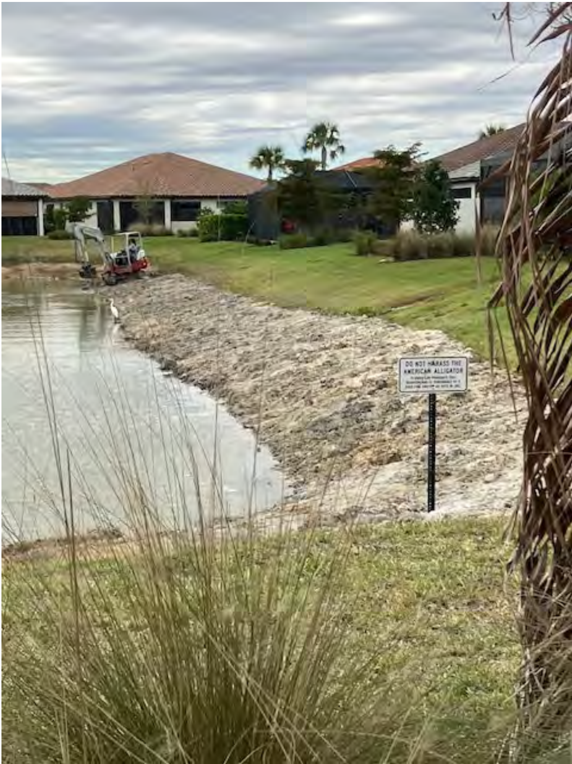
Lake bank restoration
