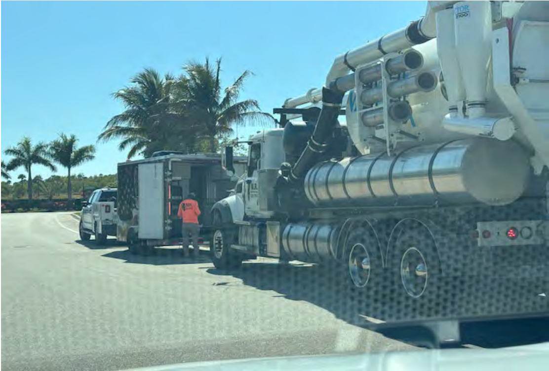
Cleaning of storm drains
