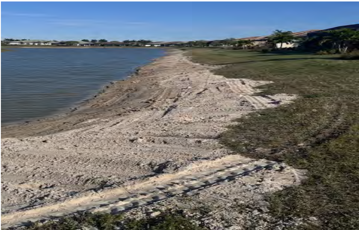
Erosion repairs on Lake 13-1
