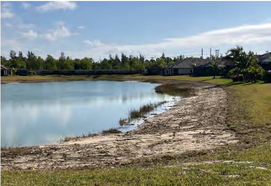
Lake bank restoration
