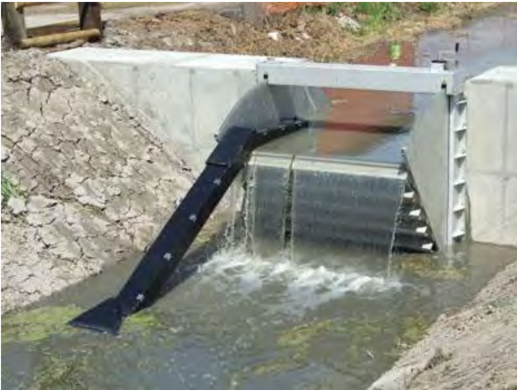
Figure 76: Other adjustable weir designs with a fish chute.
