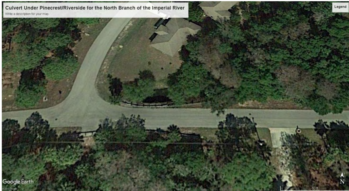
Figure 85: Culvert under Pinecrest/Riverside of the North Branch of the Imperial River
