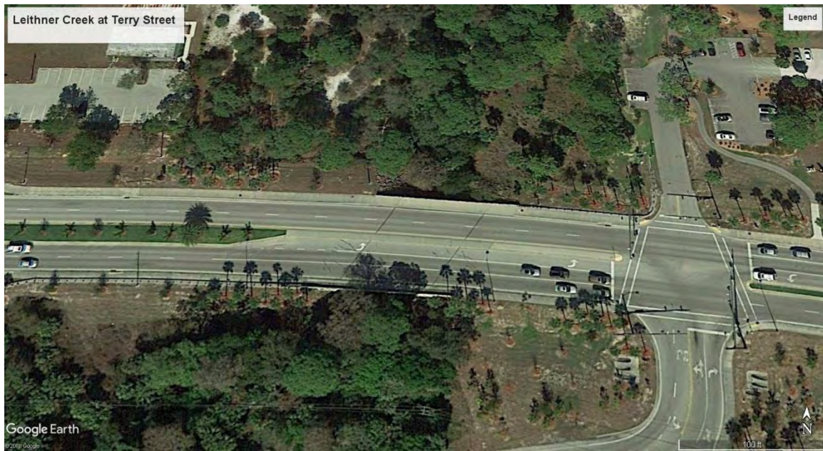
Figure 91: Leitner Creek culvert crossing at Terry Street
