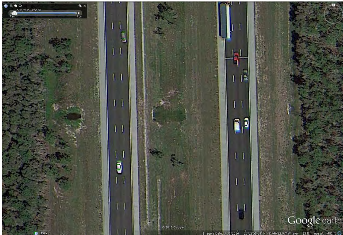
Figure 107: Culvert between Flint Penn Strand (Edison Farms) and The Brooks crossing under Interstate 75.
