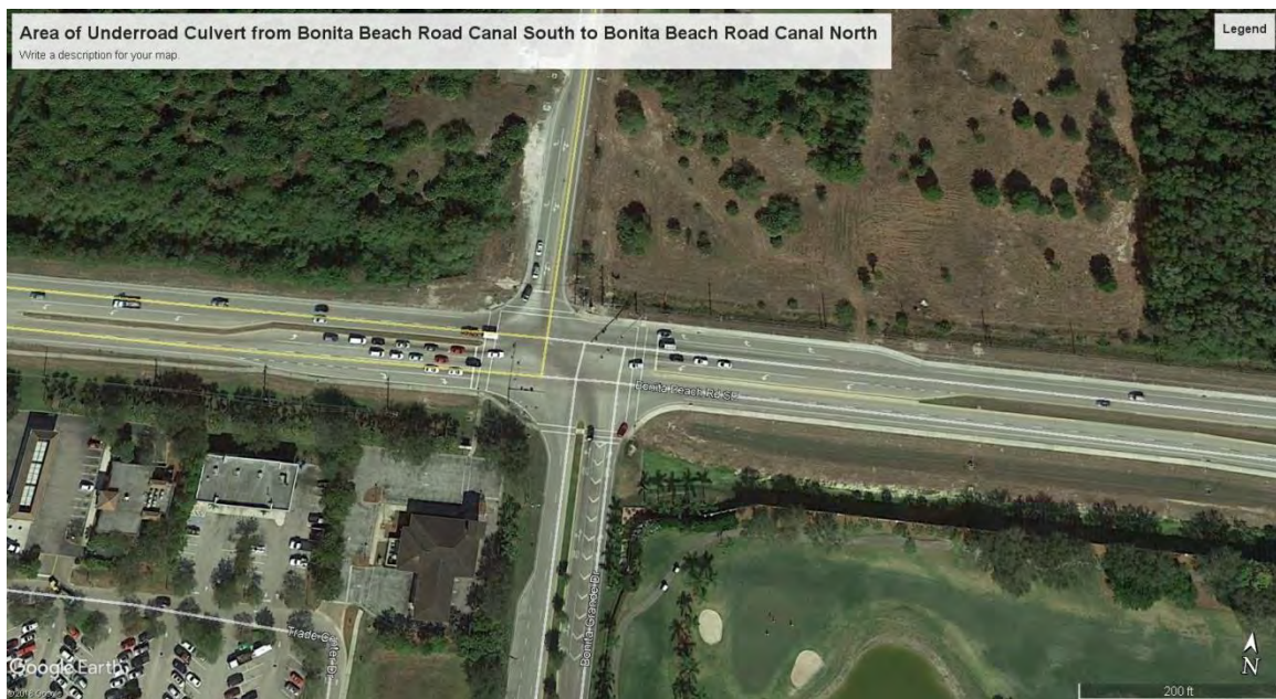
Figure 80: Bonita Beach Road Culvert Undercrossing
