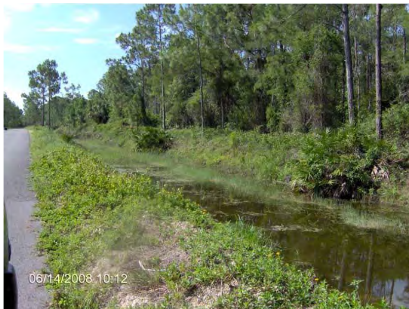
Figure 41: San Carlos Estates berm and canal system.
