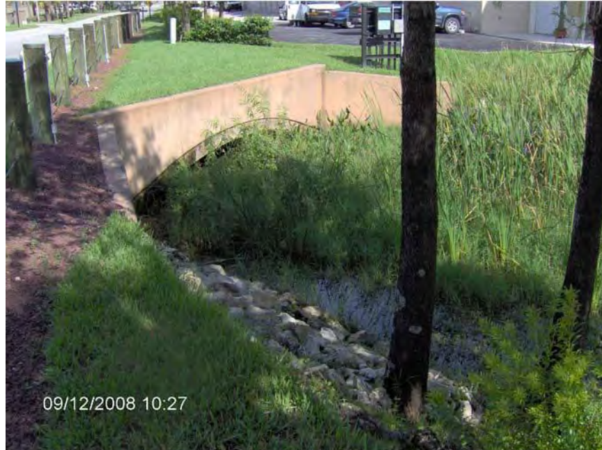
Pic 20. Culvert in Bernwood Business Park – North Branch
