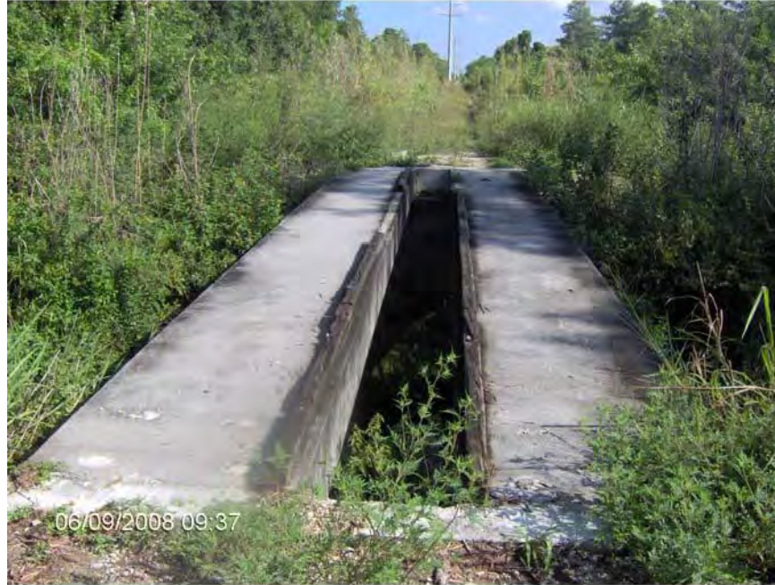
Pic 17. FPL Easement Bridge Crossing
