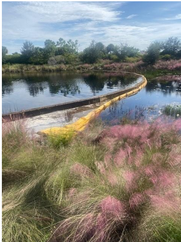
SWM - Flow Way Weir (South)
