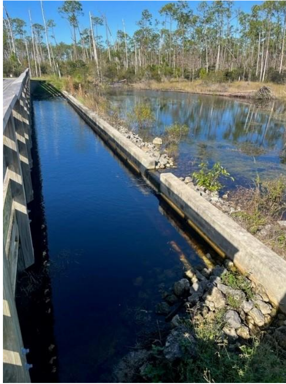
SWM - Flow Way Weir (North)
