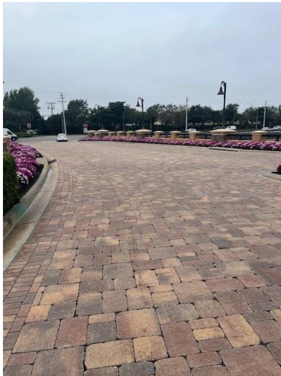
Entrance - Roadway & Lighting
