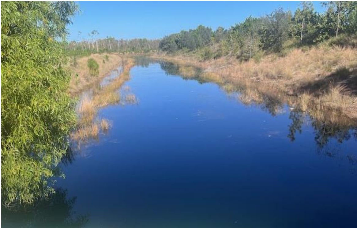
SWM - Flow Way Canal
