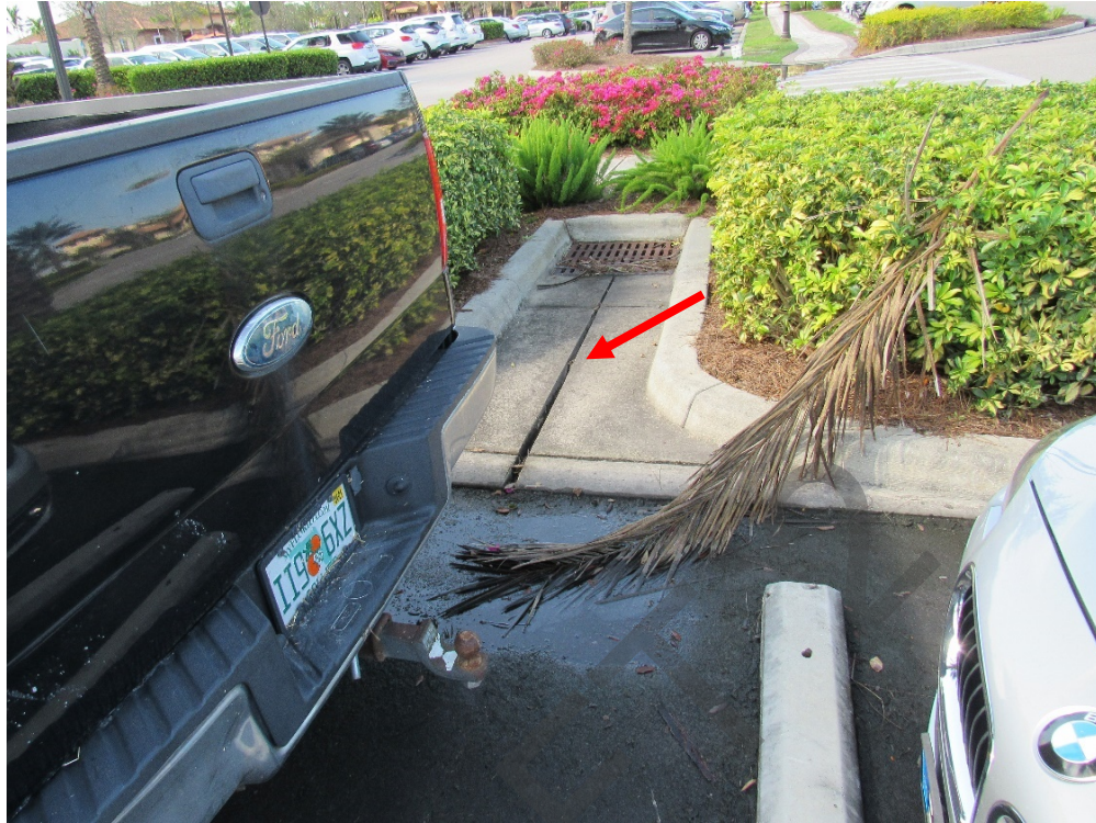
View of groove cut into concrete catch basin – Amenity Center Parking Lot.
