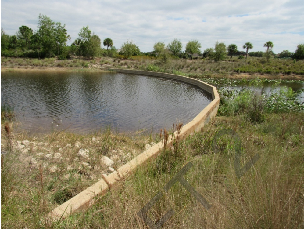
View of South Broad Crested Weir.
