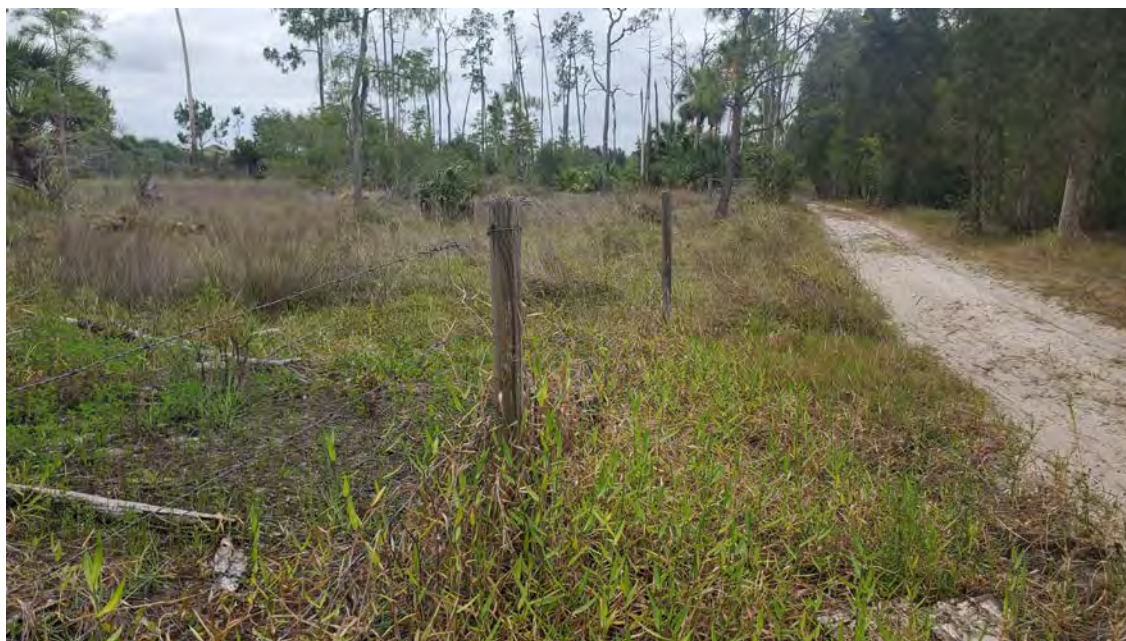
#74 - Collier ROW – Ex. Fence Terminal
