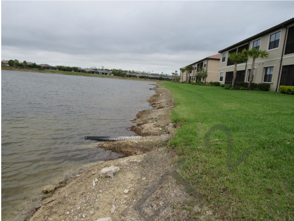
View of limited littoral plants and erosion at lake embankment - Lake 20.
