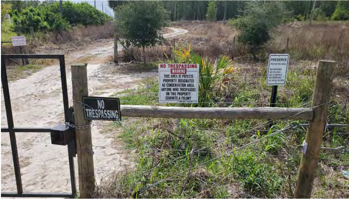
NW Logan Access – Parkland Preserve Gate & Flow Way CDD Missing Gate
