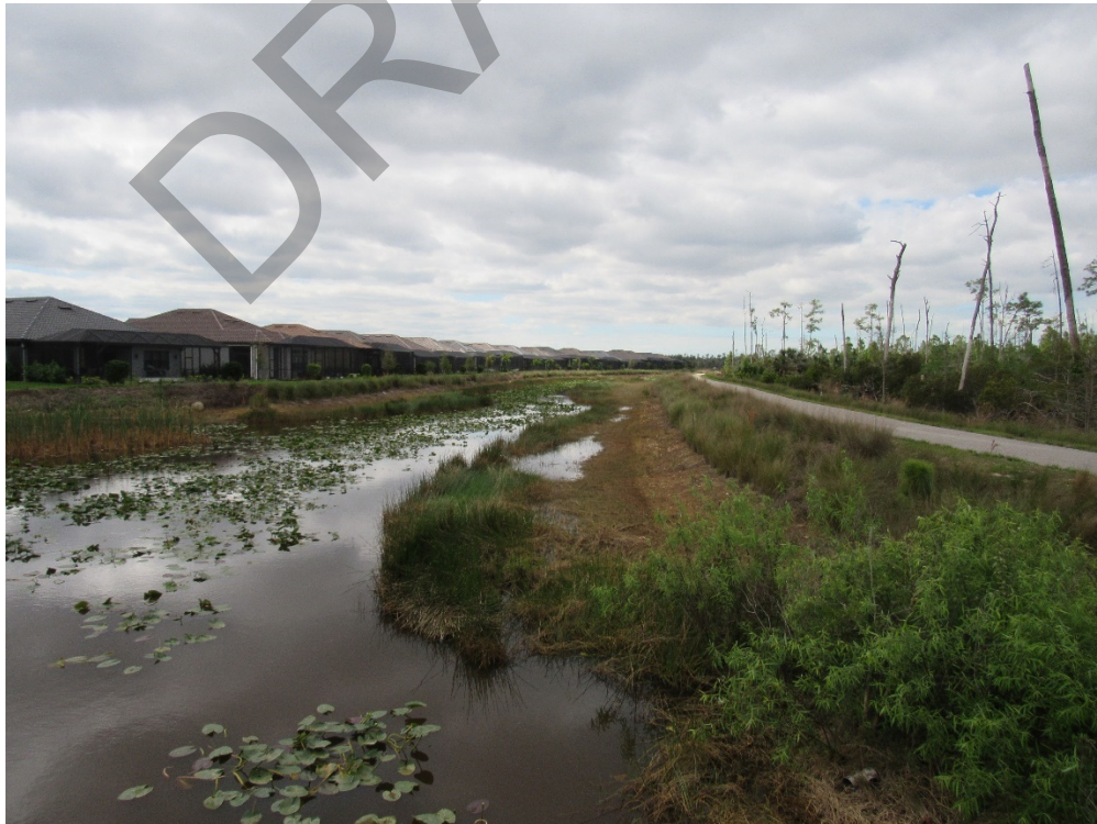
Typical view of Flow Way.
