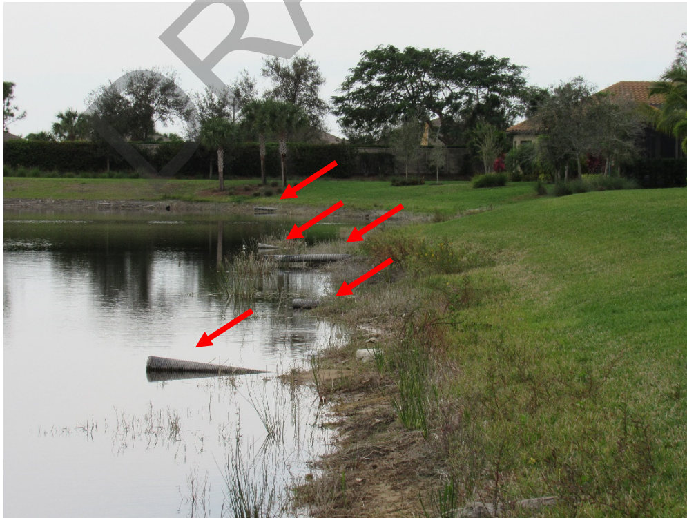
View of direct discharge lines - Lake 27.
