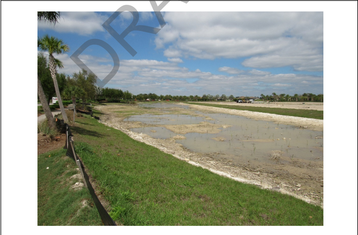
View of lake under construction - Lake 11.
