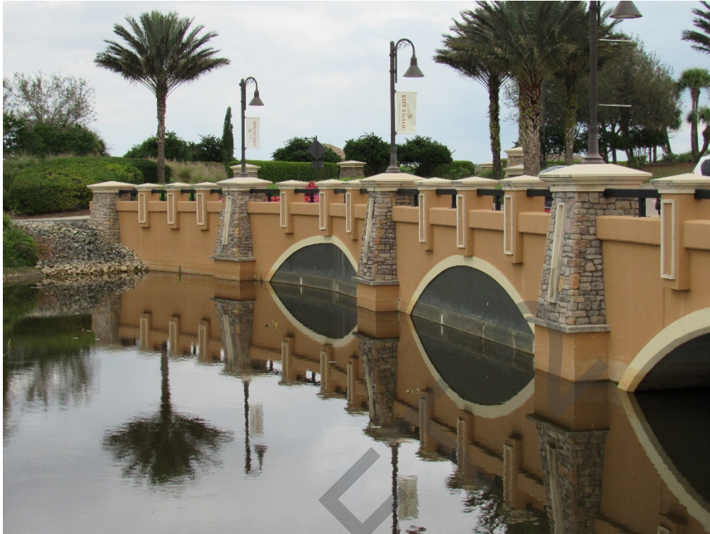
View of Entry Bridge
