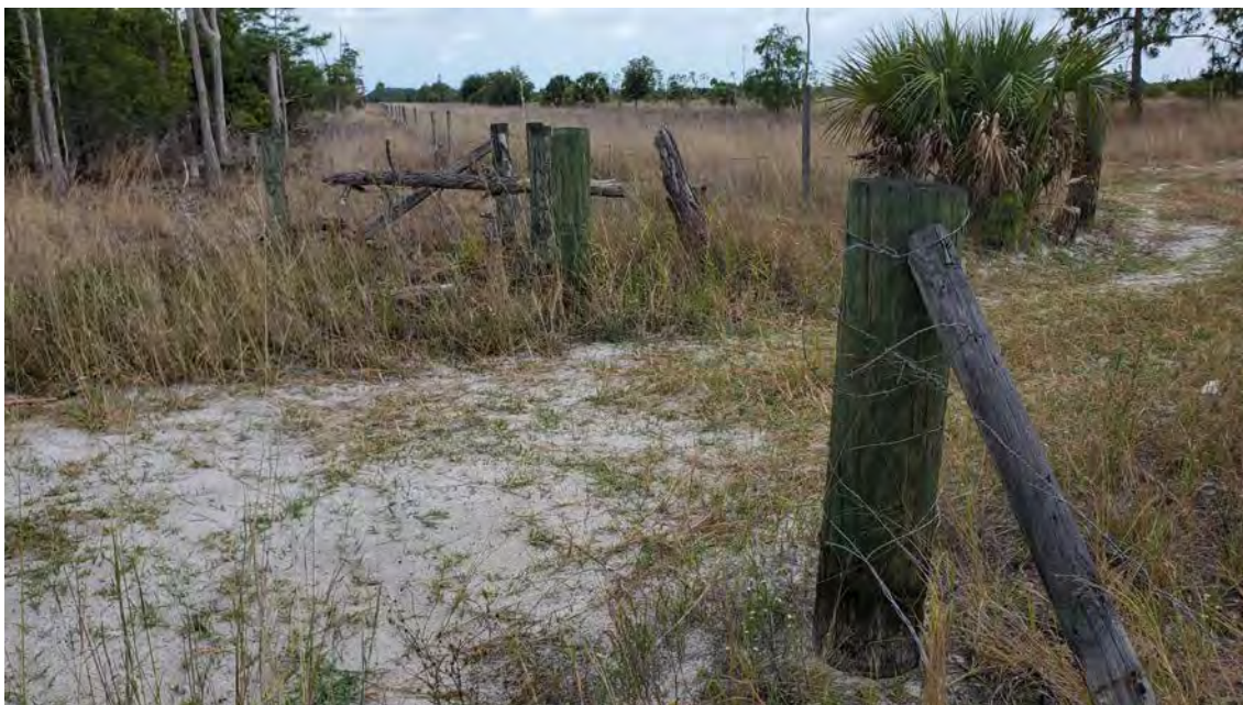
Flow Way CDD Gate 2 – Broken
