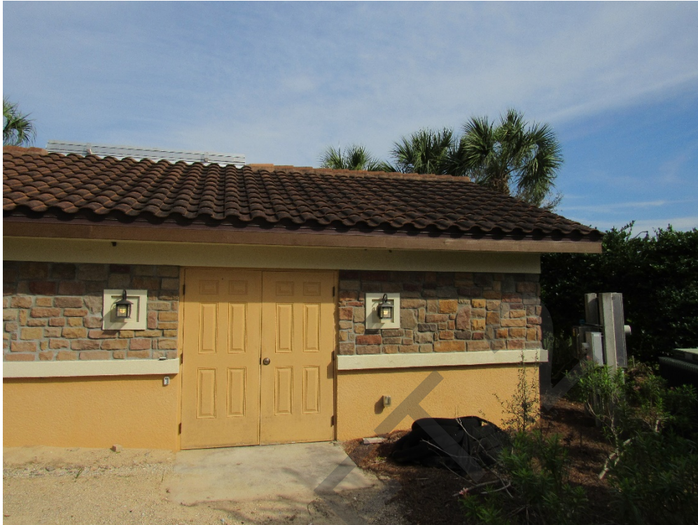
Exterior view of Community Irrigation Pump House.
