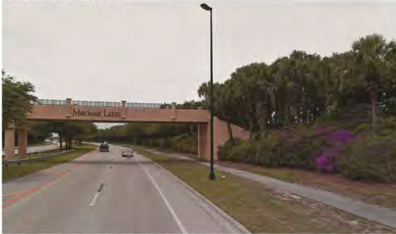
View looking south on west side of bridge.
