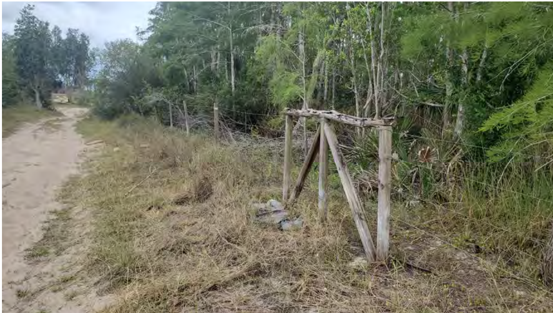
#73 - Collier ROW – Ex. Fence Good Condition
