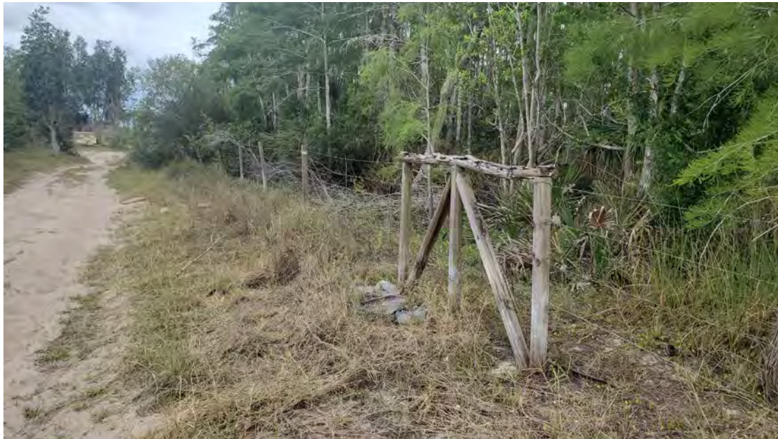
Collier ROW – Ex. Fence Good Condition
