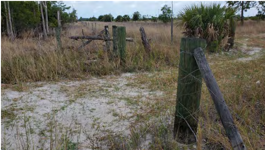
Flow Way CDD Gate 2 – Broken
