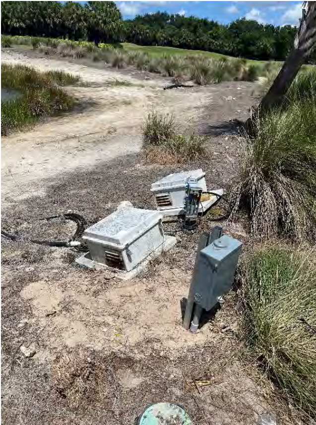
Repaired aeration power supply
