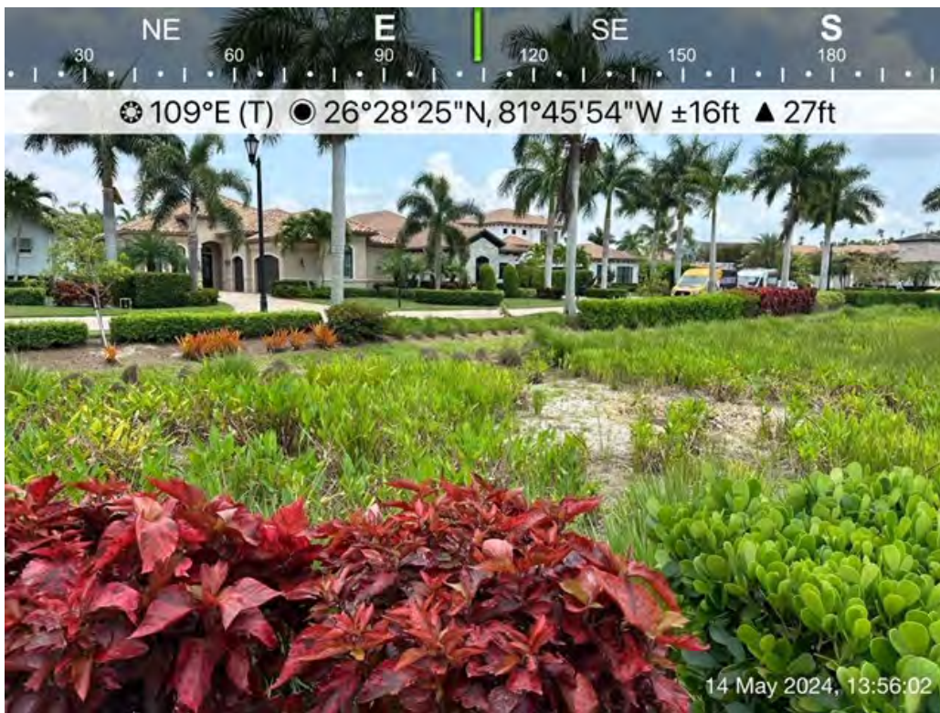
Detention area in Lugano - well maintained and clear of debris
