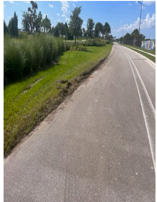
Bollard that needs to be repaired on Lorrain Blvd.
