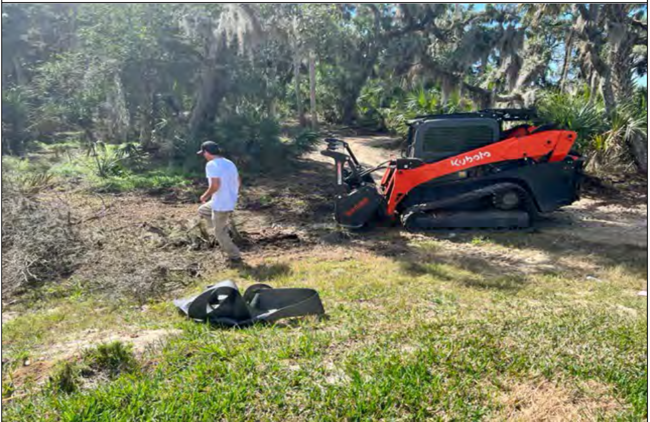
Clearing Of Debris On Shell Path
