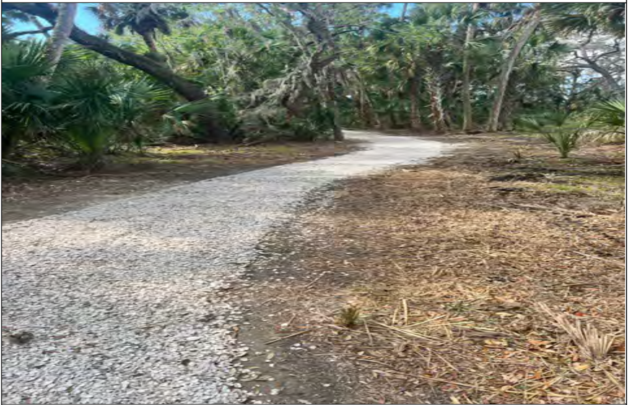
Shell Path Restored
