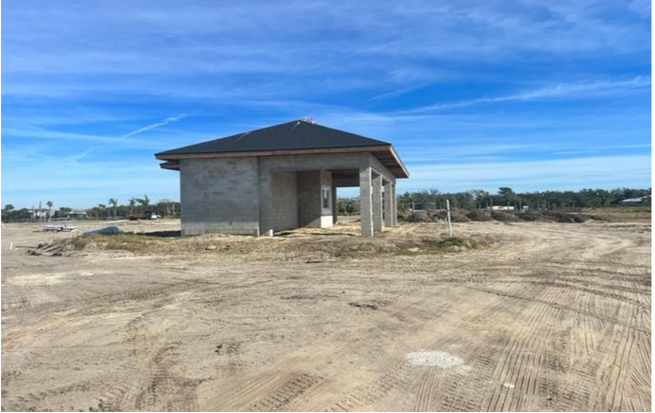
Restroom & Snack Shack
