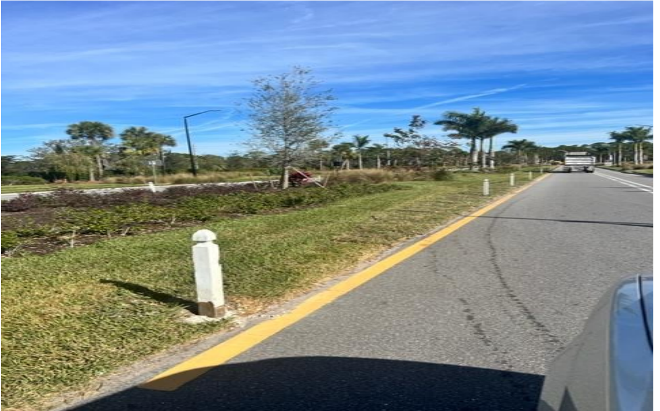
A Rut Repair on Lorraine Blvd.
