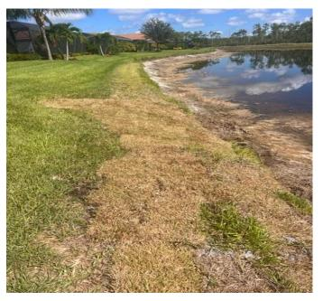
Washout on lank bank before repair
