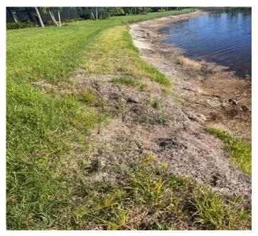
Washout on lank bank before repair
