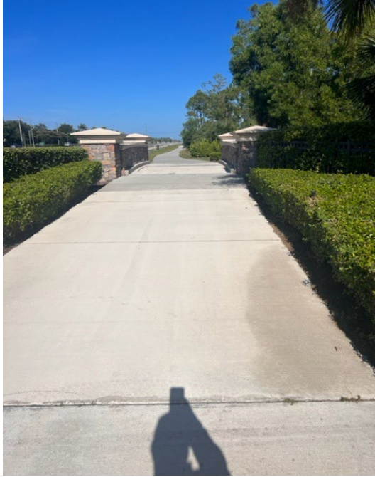
Sidewalk along the east and west entrance after being pressured washed.
