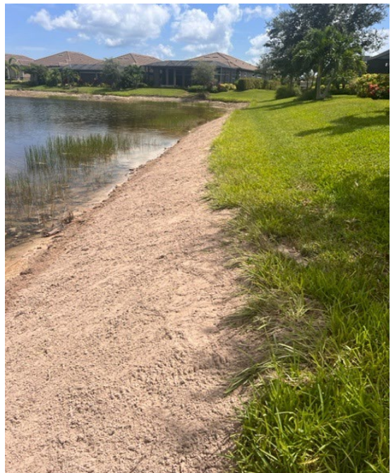
Lake bank slope regraded.
