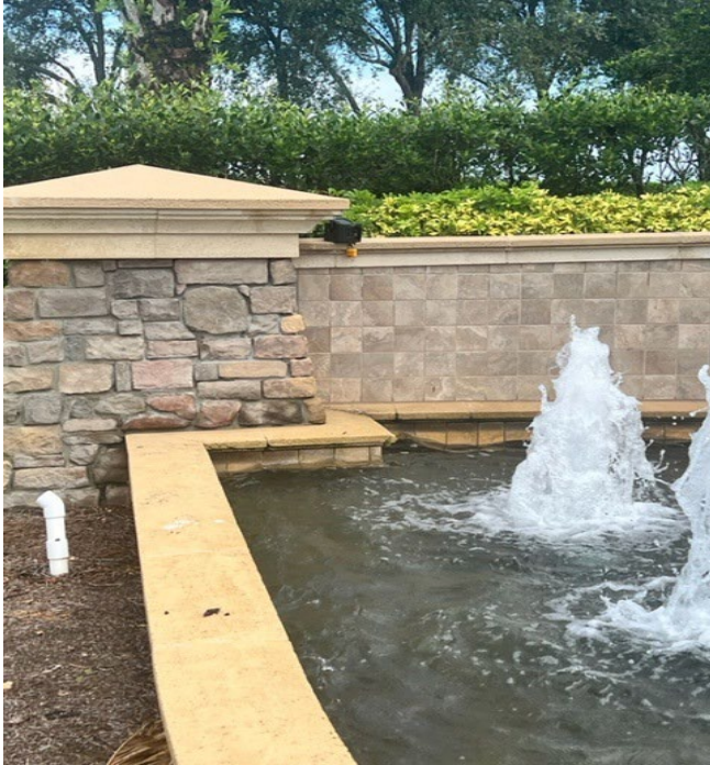
Camera installation at the fountain.
