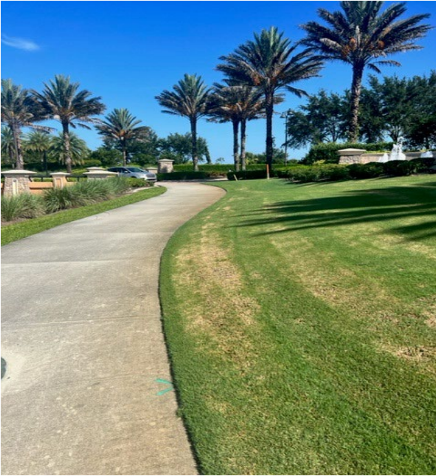
Sidewalk before it was pressure cleaned.
