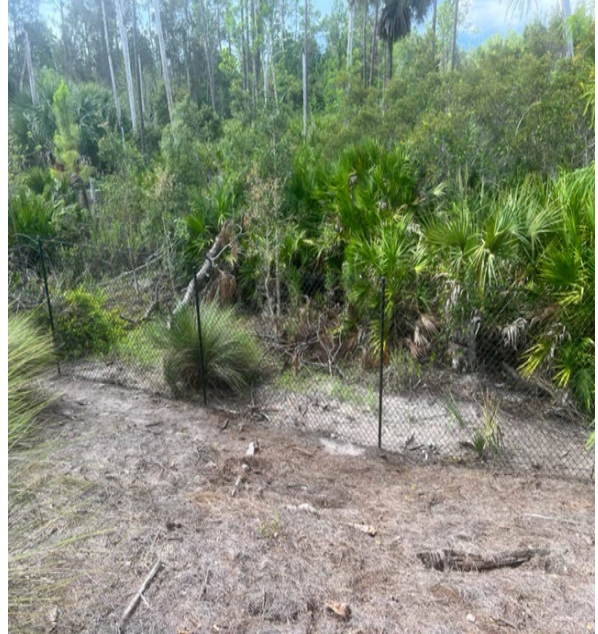
Perimeter fence repaired at Nature Trail.
