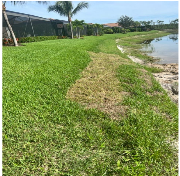
Lake Bank erosion repair.
