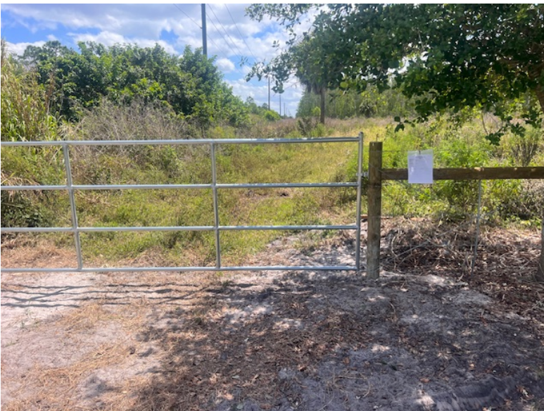
(5) Gate installation in preserves area
