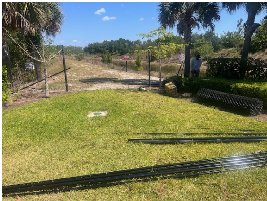
(2) New fence and gate on Immokalee Road Property Line
