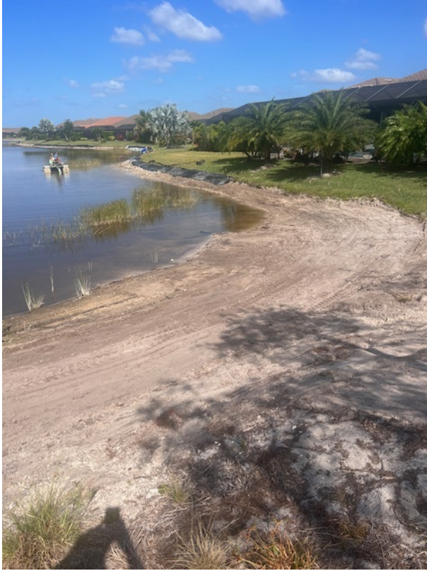
(6) Lake bank restoration on Lake 17
