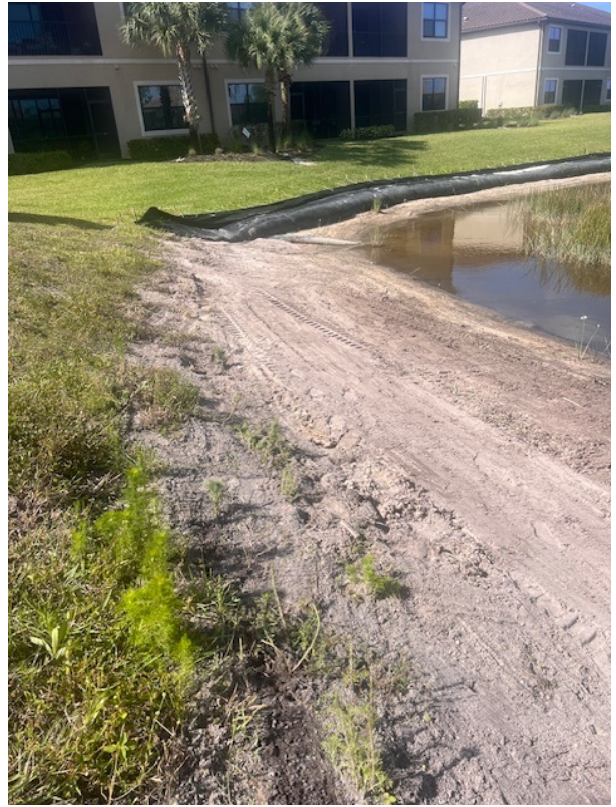
(7) Lake bank restoration on Lake 17
