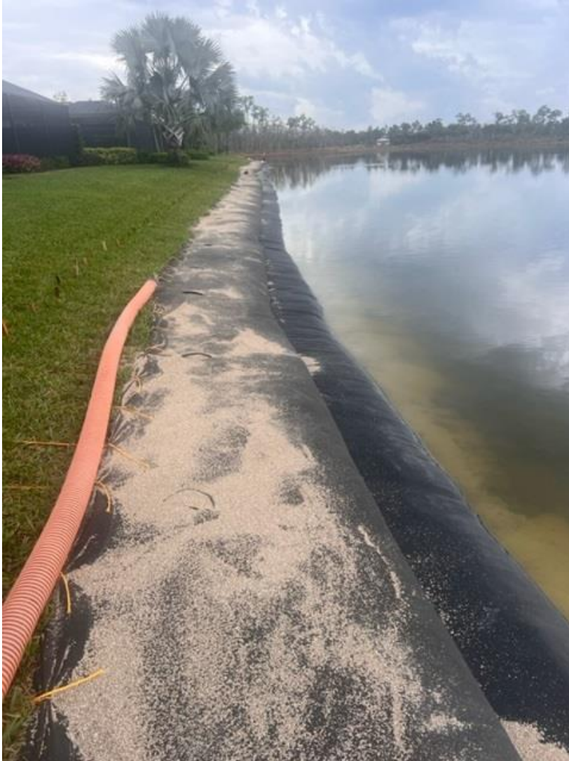
Geotube installation (in progress).
