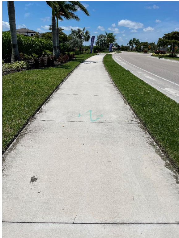
Center Place Blvd sidewalk edging.
