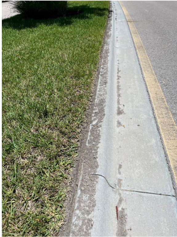
Median on Center Place Blvd being edged.
