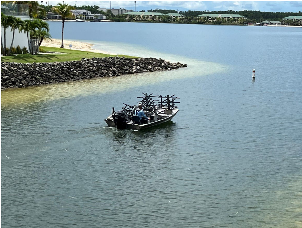
Structures being installed.
